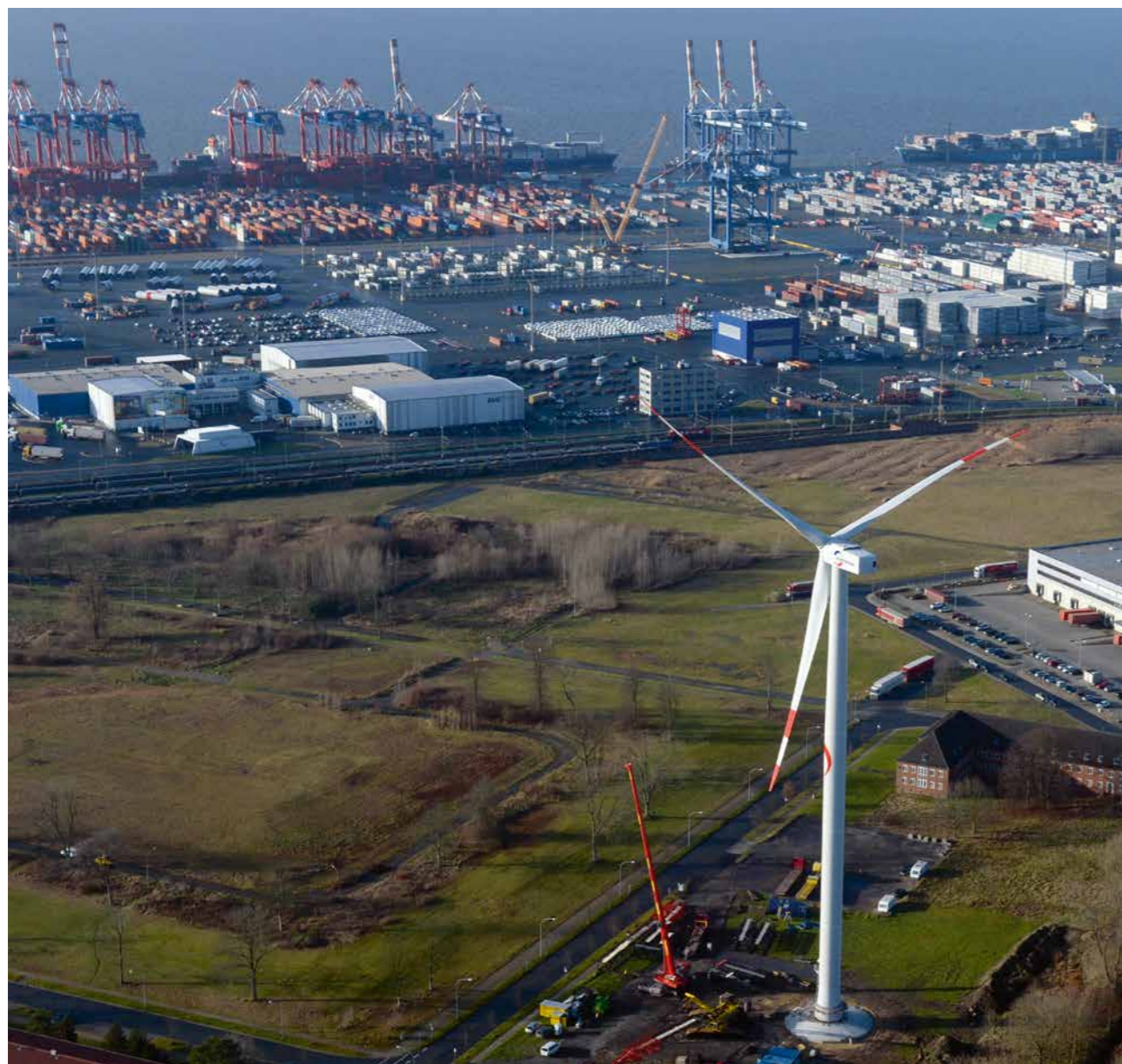
A pioneer in energy management: EUROGATE's second wind turbine stands in Bremerhaven.
