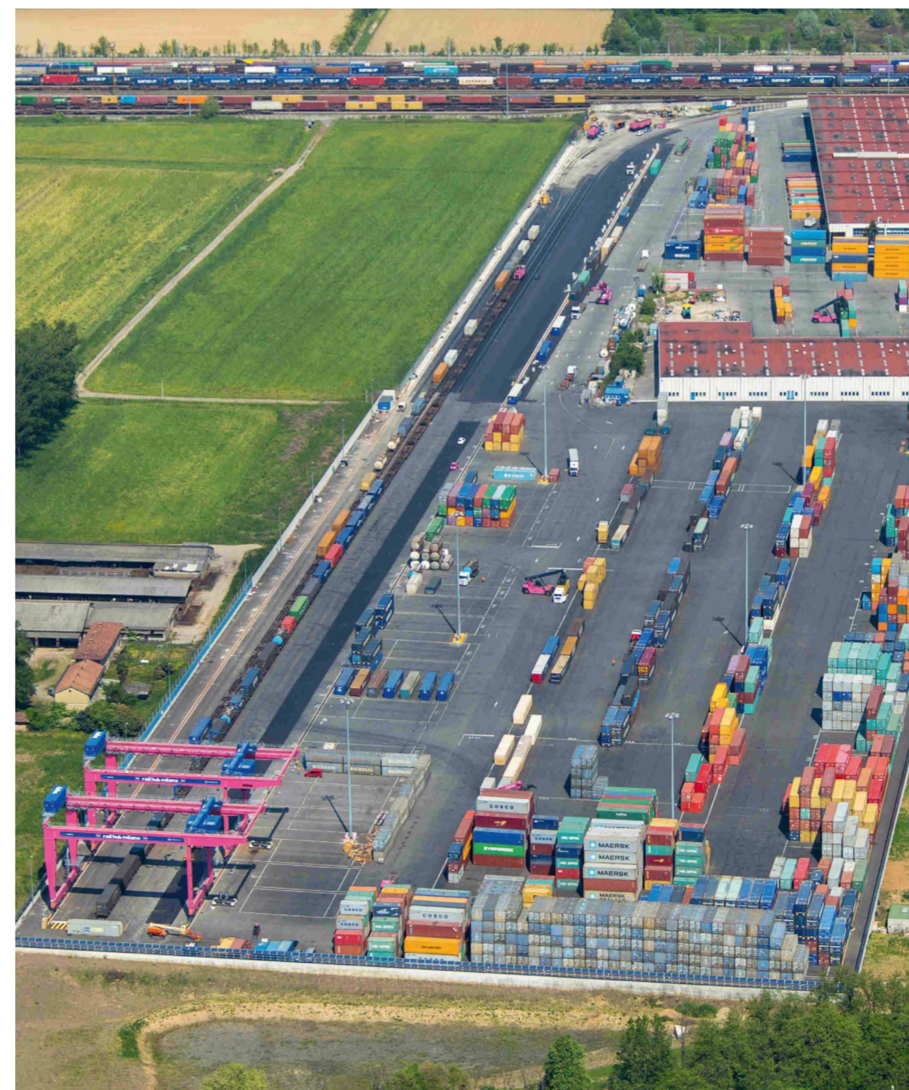
The transport node for rail transports between the Italian seaports and North and Central Europe: Rail Hub Milano in Melzo near Milan.
