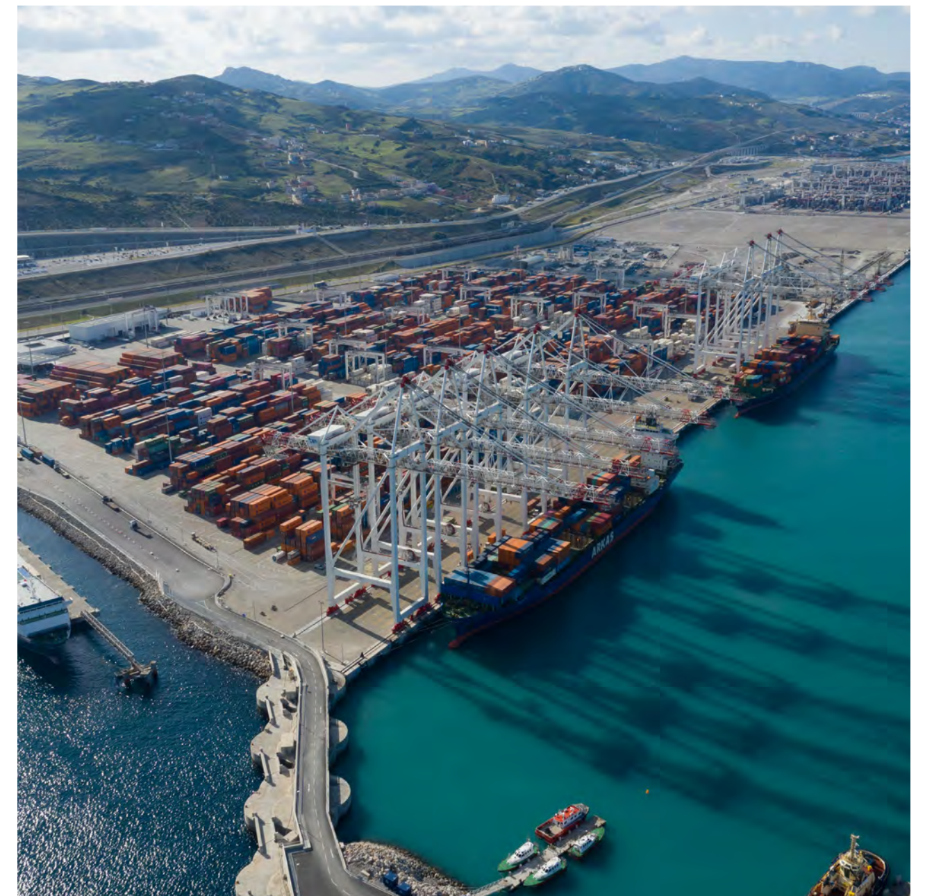
Tanger Alliance Terminal, Morocco
