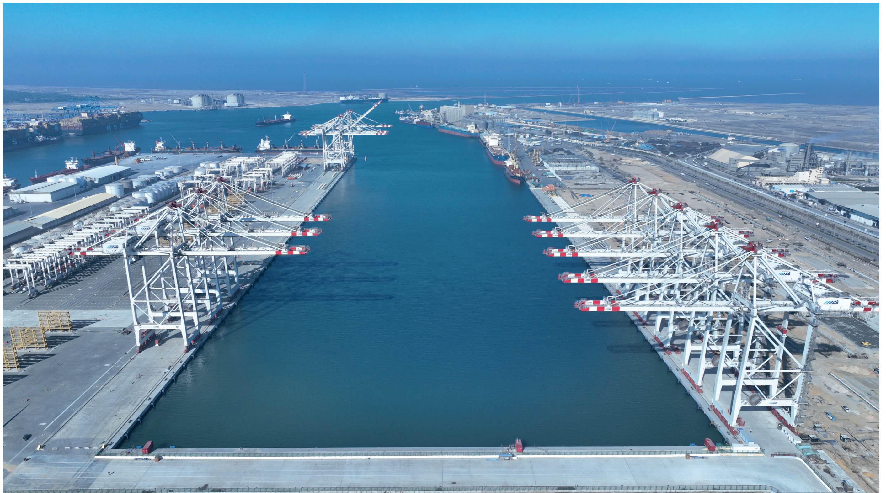
On 14 February 2026, the Damietta Alliance Container Terminal officially started its operations.
